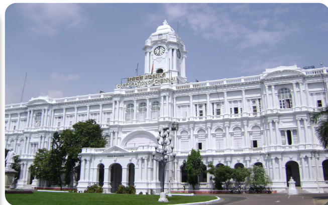
Chennai Corporation (Rippon Building)
